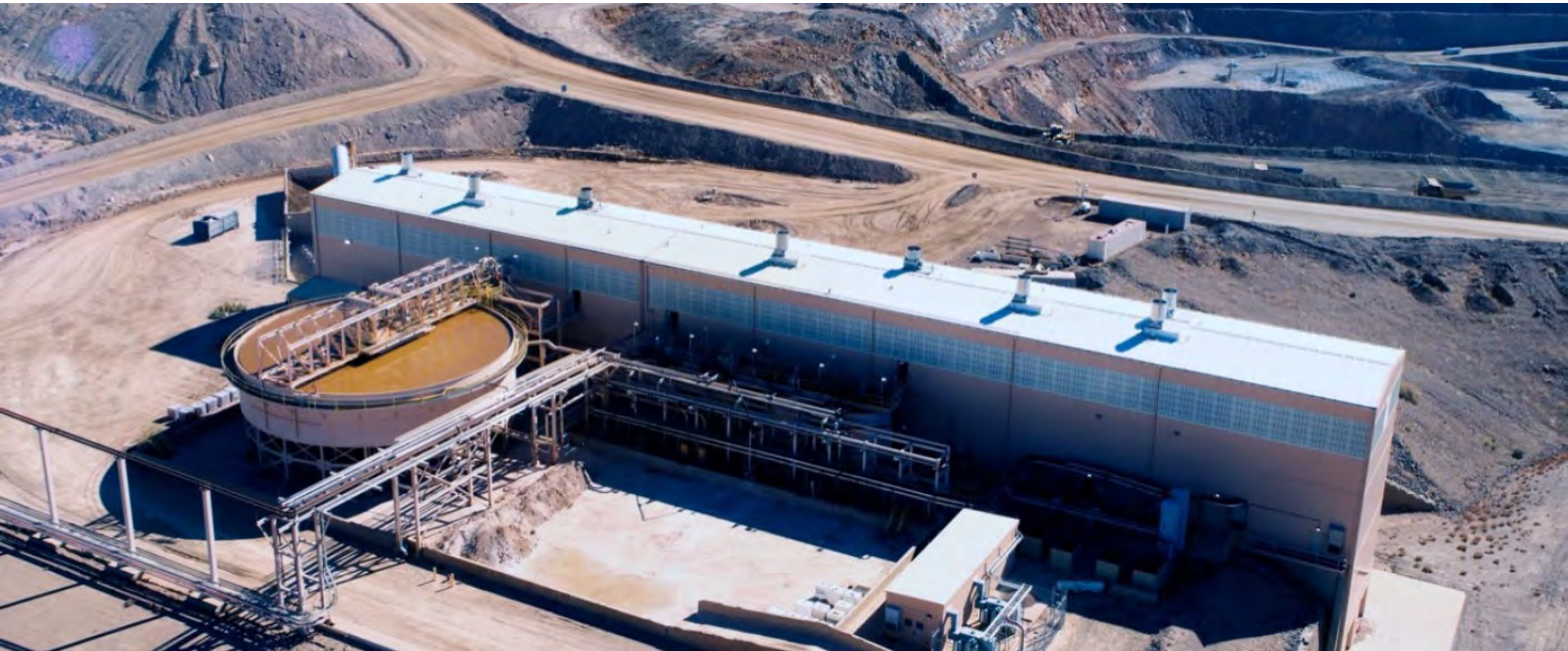
Water Reclamation Facility - Enabling sustainable water usage
